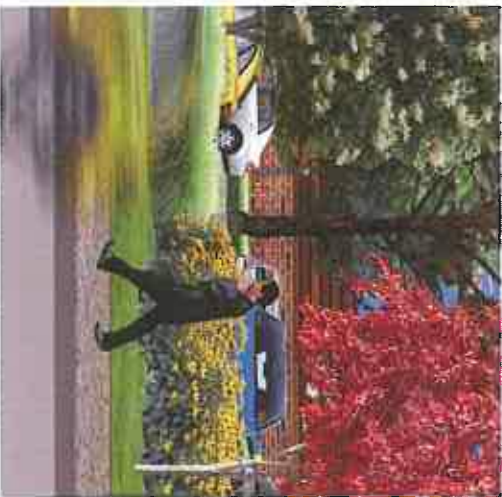
10' HEIGHT WOOD & MASONRY PERIMETER FENCE
